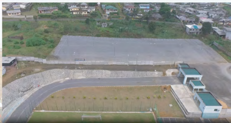
VUE PARTIELLE DU PARKING PARTIAL VIEW OF THE PARKING ZONE
