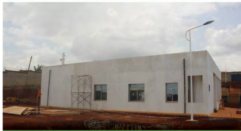
VUE PARTIELLE DES BUREAUX PARTIAL VIEW OF THE OFFICES
