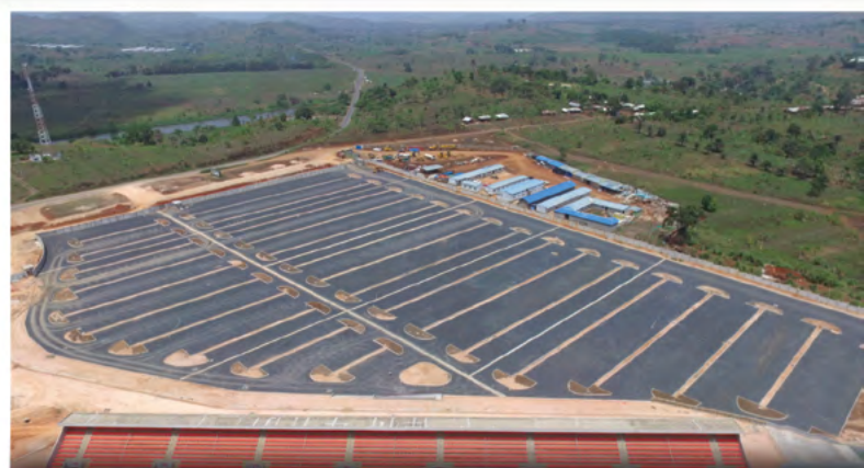
VUE PARTIELLE DU PARKING - 2080 PLACES PARTIAL VIEW OF THE PARKING ZONE - 2080 SEATS
