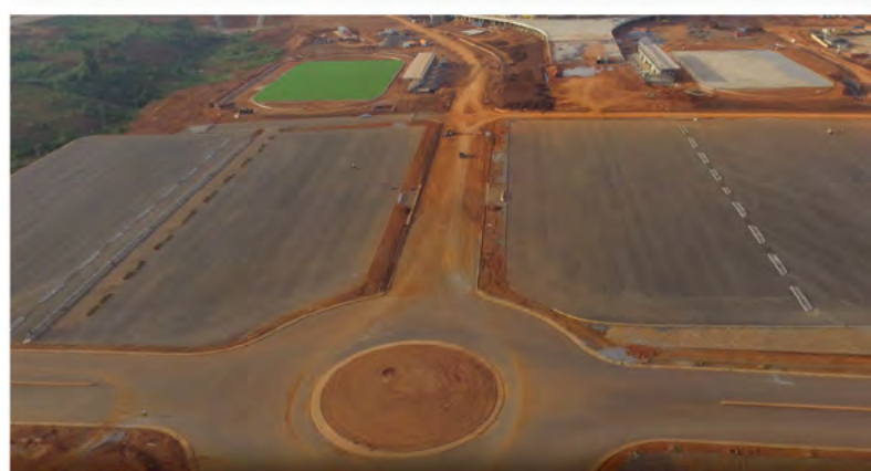
VUE PARTIELLE DU PARKING PARTIAL VIEW OF THE PARKING ZONE
