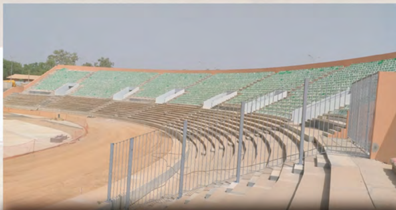
VUE PARTIELLE TRIBUNES PARTIAL VIEW OF THE TRIBUNES
