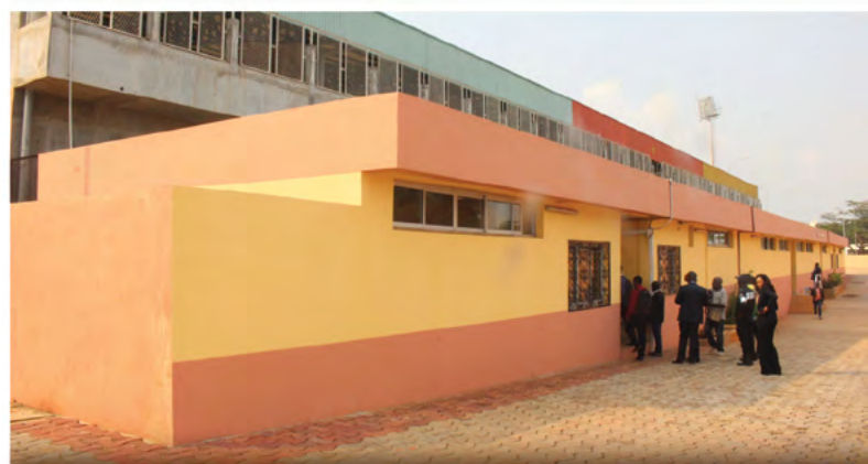
VUE PARTIELLE DES BUREAUX PARTIAL VIEW OF THE OFFICES
