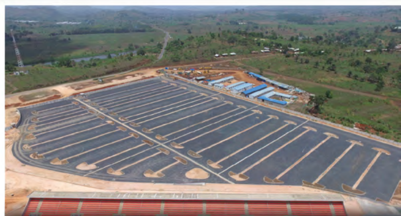
VUE PARTIELLE DU PARKING - 2080 PLACES PARTIAL VIEW OF THE PARKING ZONE - 2080 SEATS
